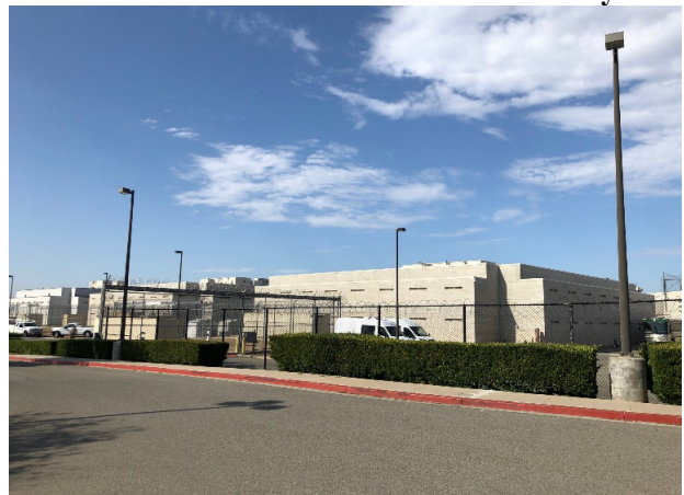
Southwest Justice Center – Jail Facility
